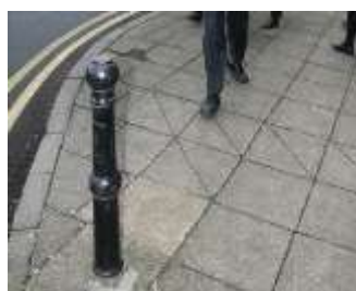
This bollard, damaged by a vehicle has now been repaired and realigned
